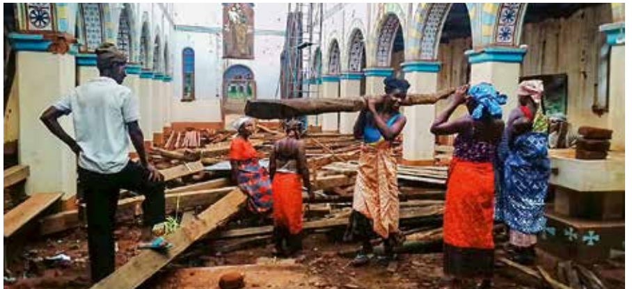
Reconstruction of St. Joseph Parish Church in Mitúcue.
